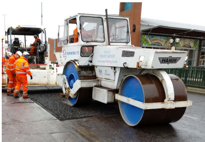
Simwhite Bridge, Frederick Ward Way
